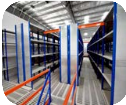
P8 Mezzanine Floor
